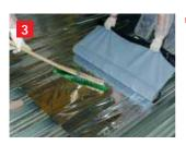
Press the edge to the profiled decking.
