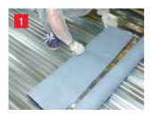
Unroll the membrane, align and set it into position along to other rolls and profiled decking.
