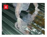
Proceed by rolling the membrane on the decking and simultaneously pulling off the siliconized film.
