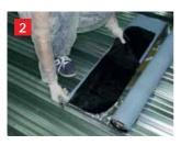
Once aligned, peel back one end of the siliconized film.
